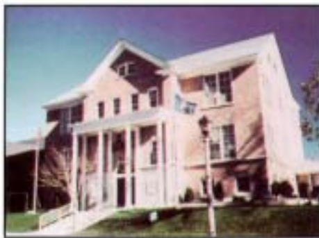
Shorewood Village Hall Architect: Kahler, Slater, Trophy, Engberg, Inc. Contractor: Double T Painting Co. Specifications included paint stripping, cleaning and waterproofing with Diedrich Chemicals
