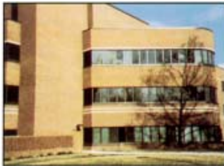
Michigan Veterans Facility — Grand Rapids, MI Architect: G.S.A. Contractor: Mercury Caulking
